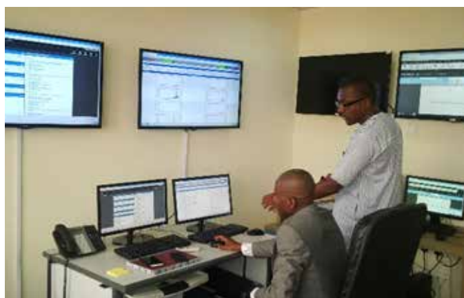
Network Operating Centre, USPF HQ, Abuja
